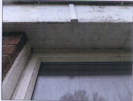
Plate 12. Ply barge board absent (flat roof)
