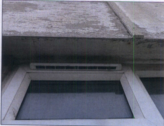
Plate 13. Ply barge board absent (pitched roof)
