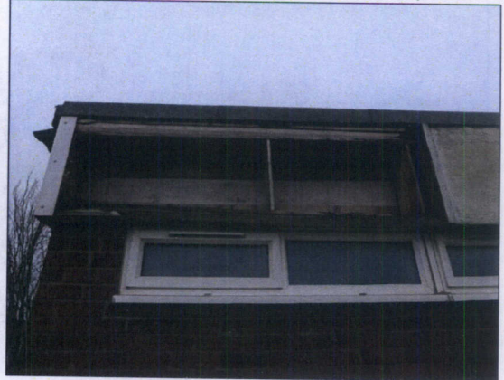
Plate 14. Flat roof covering flush to fascia boards
